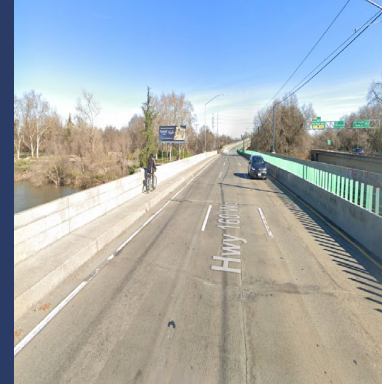
State Route 160 Bridge
