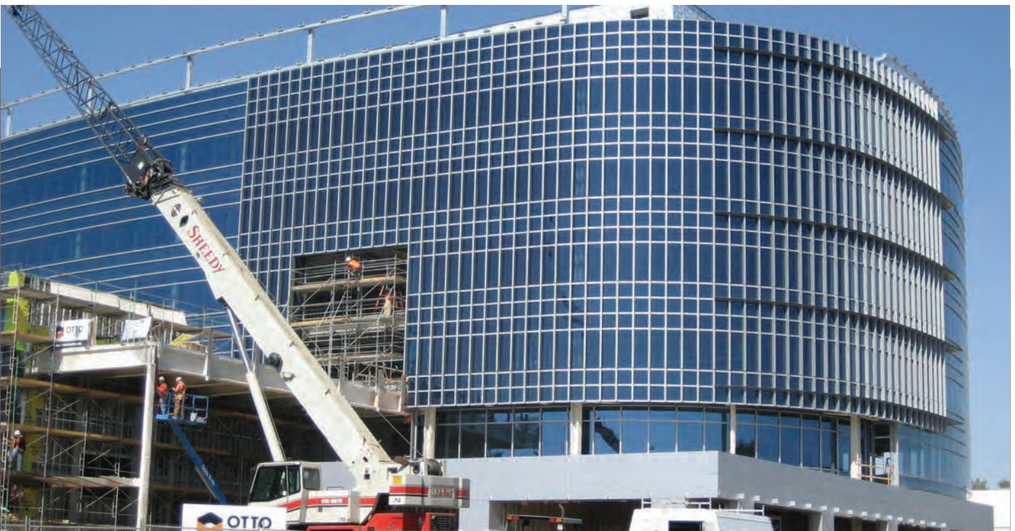
FIGURE 3.0 Lottery Headquarters under Construction, 2010.
