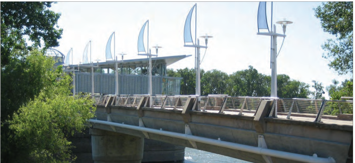
FIGURE 2.0 Sacramento River Water Intake Facility.
