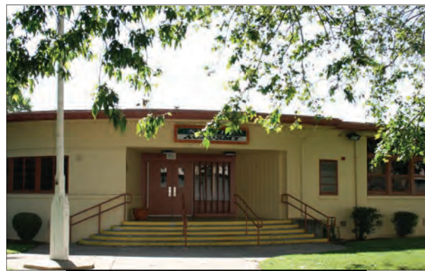
FIGURE 3.10 Former Dos Rios Elementary School, Now Smythe Academy.
