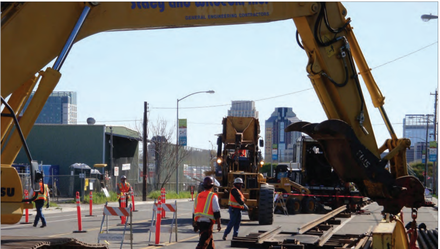
FIGURE 9.0 Light Rail Lines Being Laid on North 7th Street for the First Stop on the Green Line.
