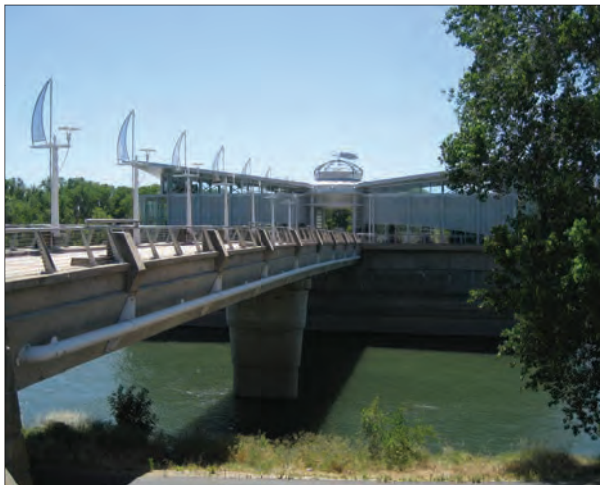
FIGURE 8.3 Sacramento River Water Intake Facility.
