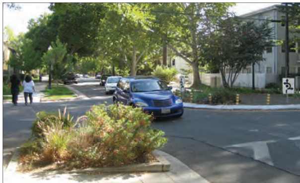
FIGURE 5.9 Traffic Circles Reduce Speeds and Provide Landscaping Opportunities.
