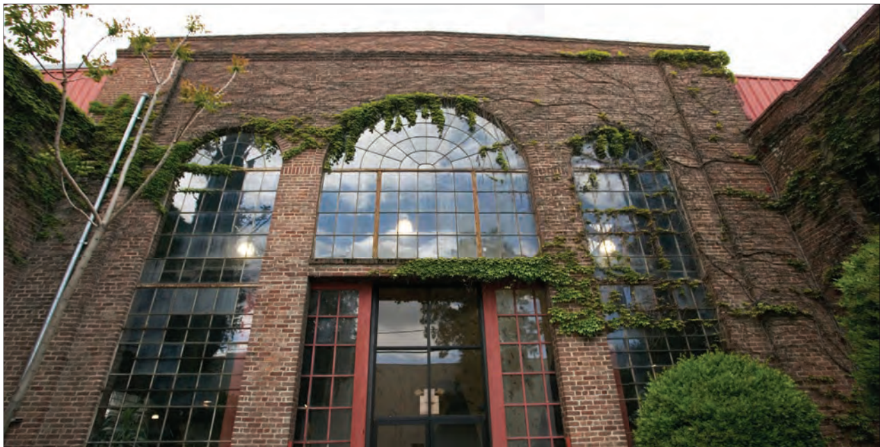
FIGURE 4.4 Pipeworks Fitness, at 116 North 16th Street.
