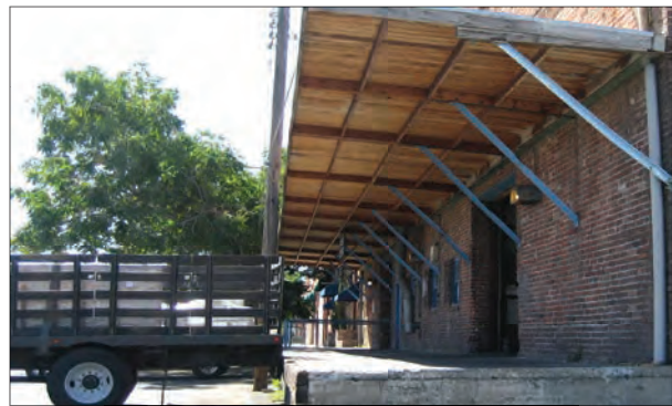
FIGURE 4.8 Elevated Docks are Common in the Historic District.
