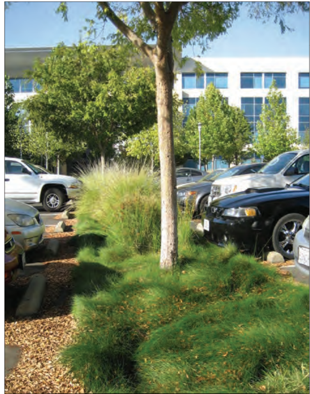
FIGURE 8.1 Example of a Bioswale.
