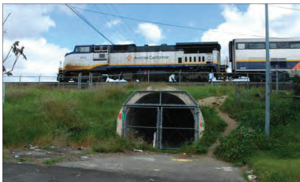
FIGURE 5.8 North 14th Street Tunnel, Closed in 1994.
