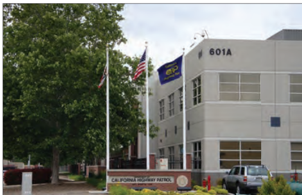
FIGURE 3.9 California Highway Patrol, Headquarters on North 7th Street.
