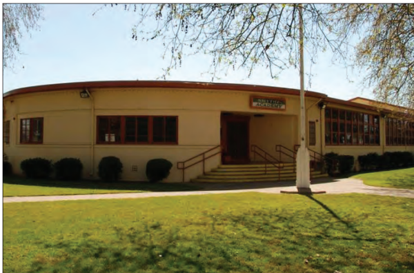
FIGURE 7.4 Former Dos Rios Elementary School, now Smythe Academy
